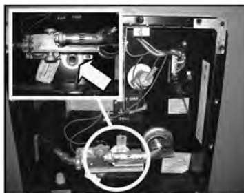
Water Heater Drain Plug Location
